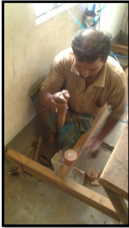
Figure 7-14: The carpenter is fixing the pulleys.
